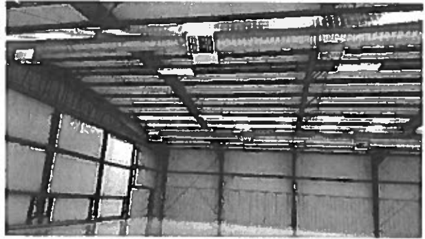
International Sunport Snow Barn Complex: interior
