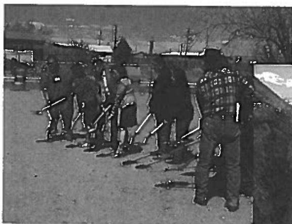
Santa Clara Pueblo Groundbreaking
