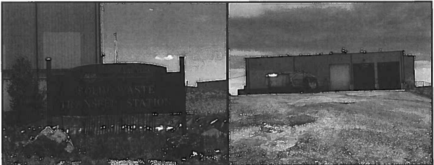
Molzen Corbin assisted the City of Las Vegas with site selection, programming, and public input for the solid waste transfer station.
