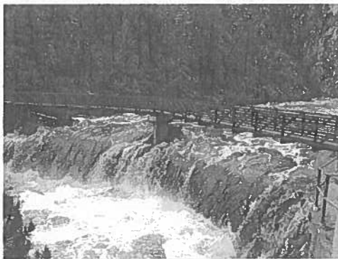
Diversion Structure During Flooding
