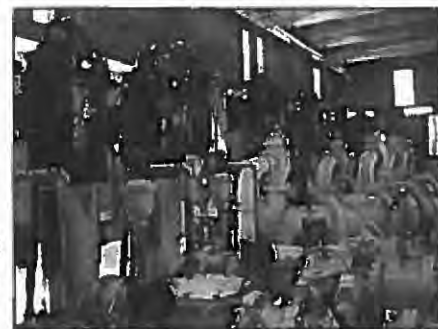
Pump structure interior, Southside Water Reclamation Facility.
