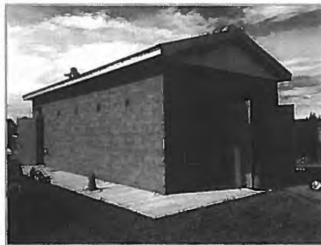
Molzen Corbin assisted the City with the North Grand Avenue Effluent Reuse Project including a 100,000 gallon water tank, booster pump station, yard piping, site work, and a jack and bore under North Grand Avenue.
