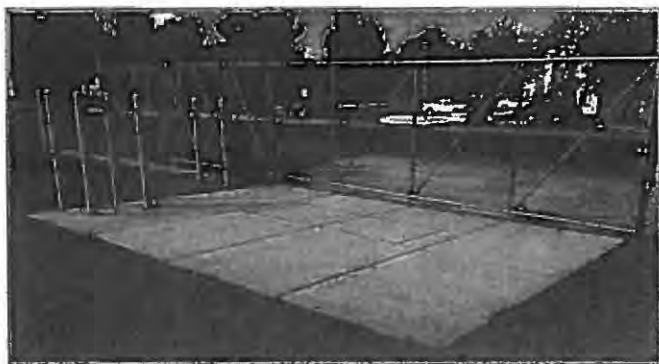
Molzen Corbin provided the design of site improvements at New Mexico State University, including an automatic gate.
