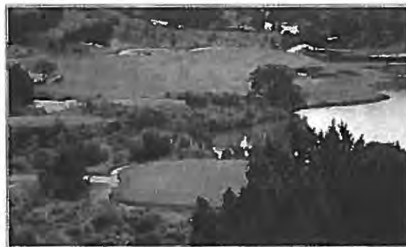
Molzen Corbin planned, designed, and provided construction phase services for wastewater treatment and disposal facilities serving the golf course community of Las Campañas near Santa Fe.
