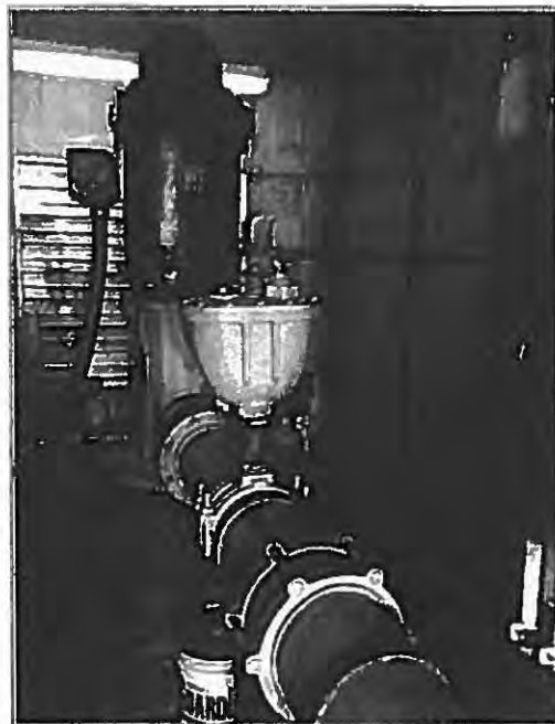
Molzen Corbin lead the Taylor Well 4 rehabilitation and pipeline project.
