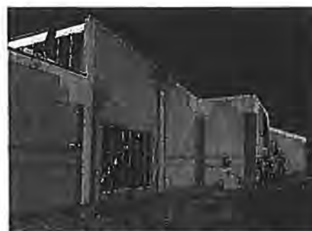
East Façade of the Abe Montoya Rec Center Renovation Project
