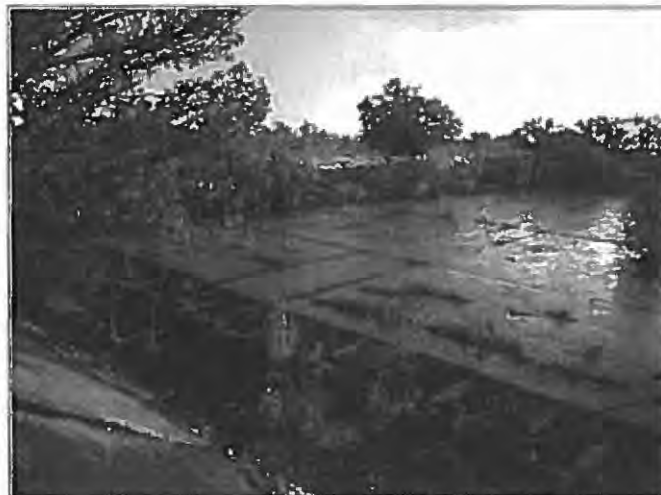
Molzen Corbin assisted the City with the Camp Luna Effluent Ponds project prior to the project being placed on hold for funding issues.
