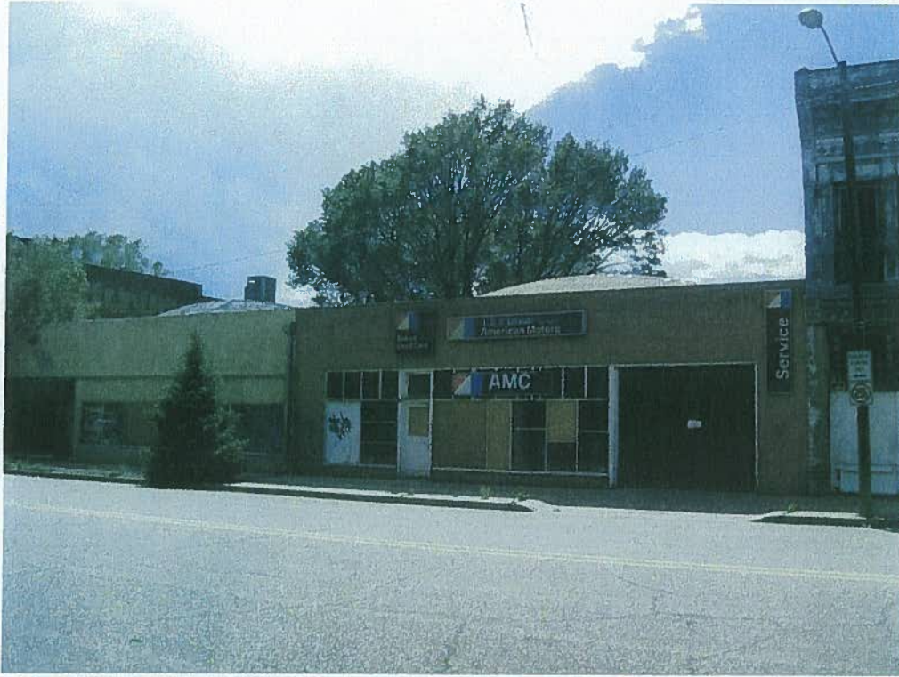
Photo 8. Ed's Motor Co. building adjacent to the south (facing west)
