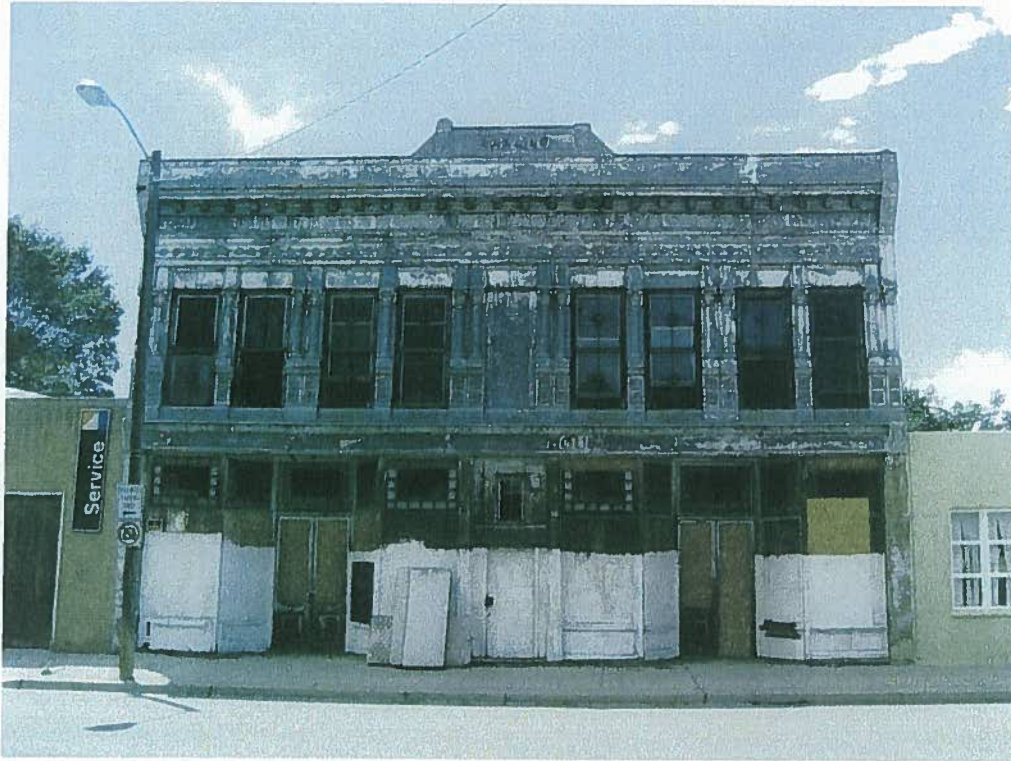
Photo 1. Rawlins Building (facing west)
