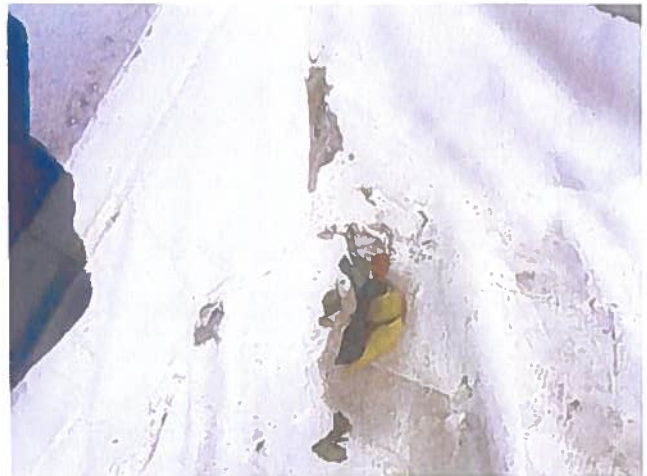
The PVC liner currently on this building has multiple breakdowns. Seems that have come apart and wear and tear.
