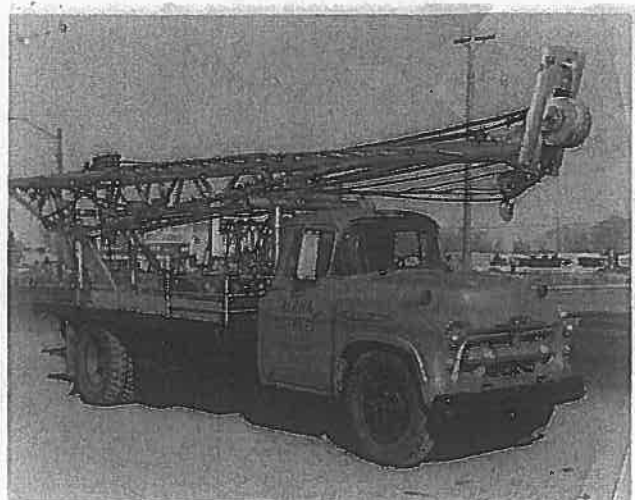
Alpha Southwest - 1964 - First Well Workover Truck
