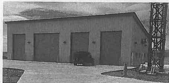
Las Vegas Snow Equipment Removal Building
