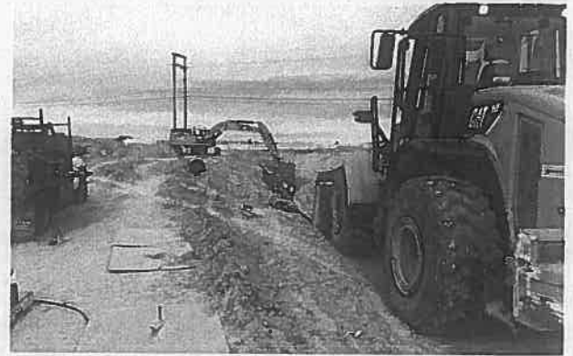
Montoyas Arroyo Sanitary Sewer Improvements CM
