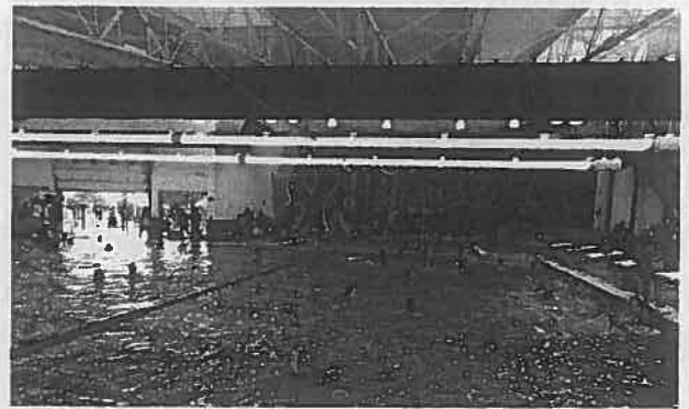
Rio Grande Swimming Pool HVAC
